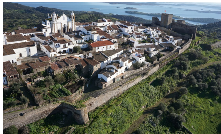
Panoramic View Previous to Project. Barbican Path. 2016 © JF
